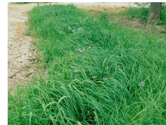
Swale planting – help with the removal of contaminant and assist in increased filtration
